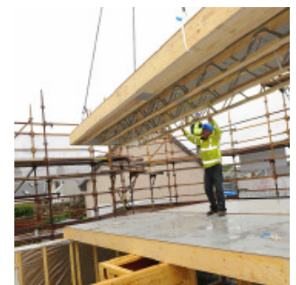
Crane Erection of Floor Panels
