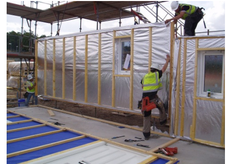
Large Panel Erection
